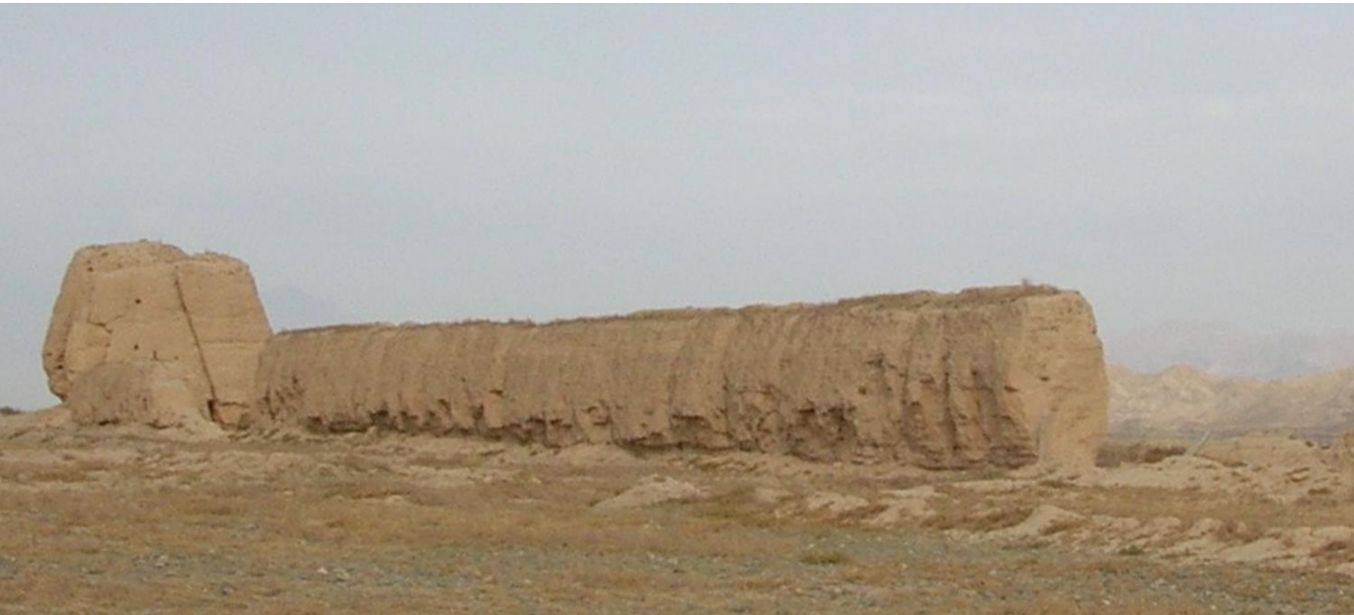
Tamarind sheets between rammed earth lifts
